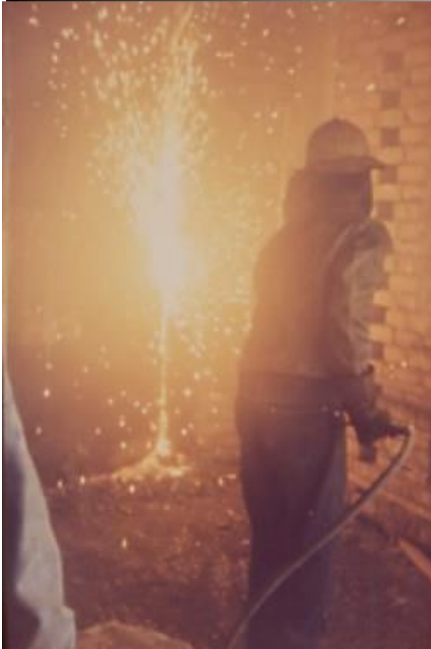
Thermal Lance in lieu of mechanical breaking, Mount Road Police Station, Port Elizabeth (Smallwood, 1987)
