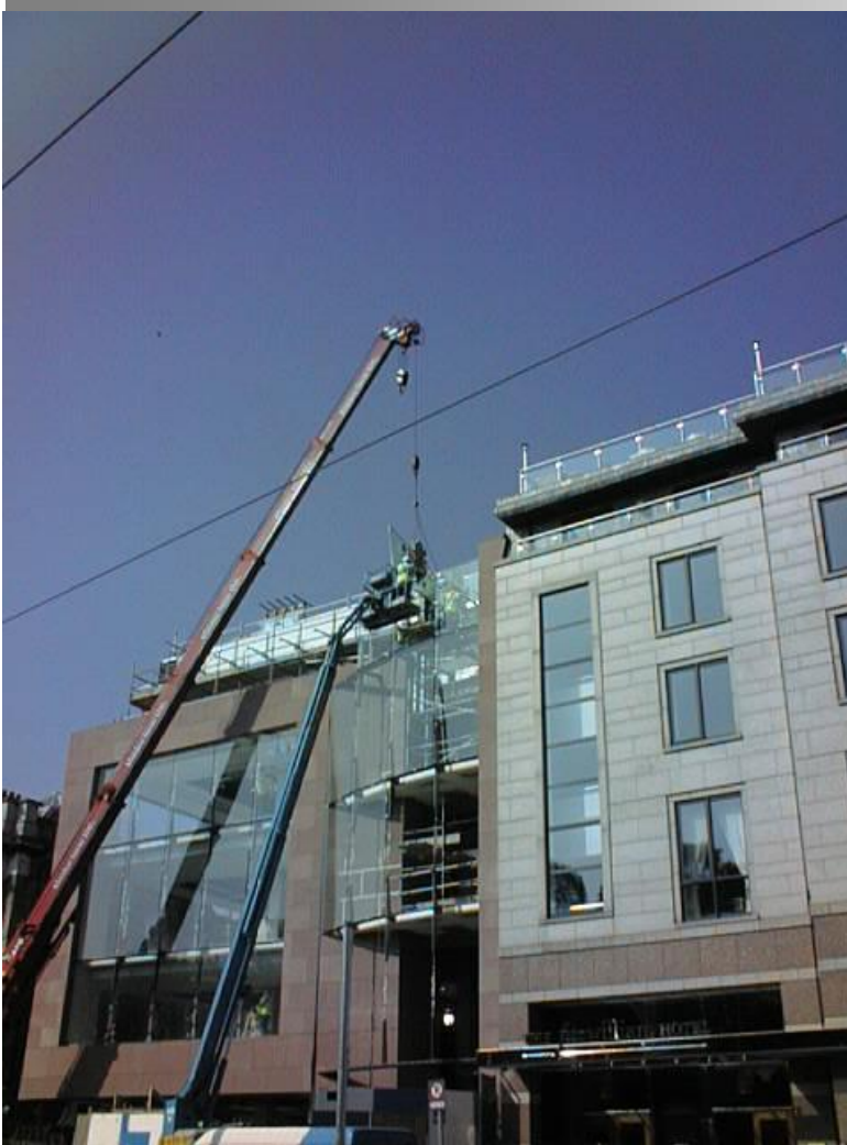
Externally installed full fenestration, Dublin (Smallwood, 2004)
