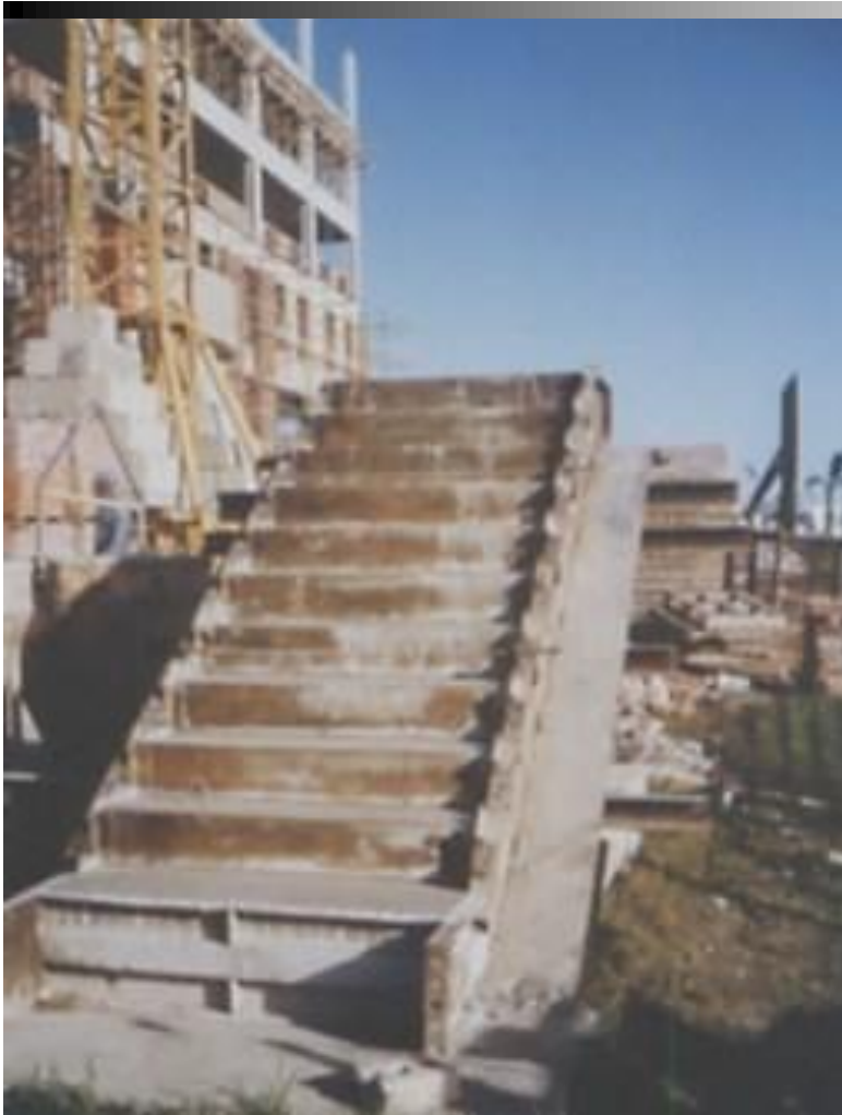
Precast concrete stair flights, Port Elizabeth (Smallwood)
