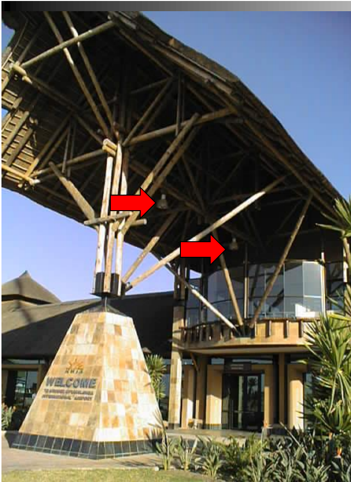
Porte Cochere, Nelspruit Airport (Smallwood, 2004)
