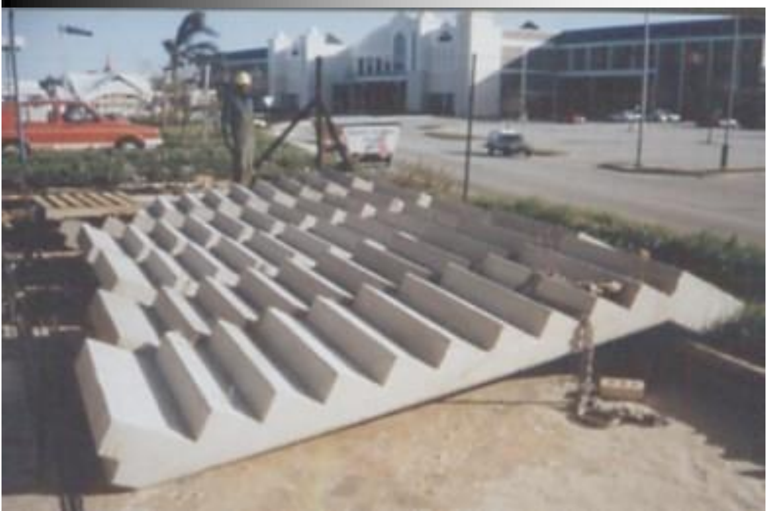
Precast concrete stair flights, Port Elizabeth (Smallwood)
