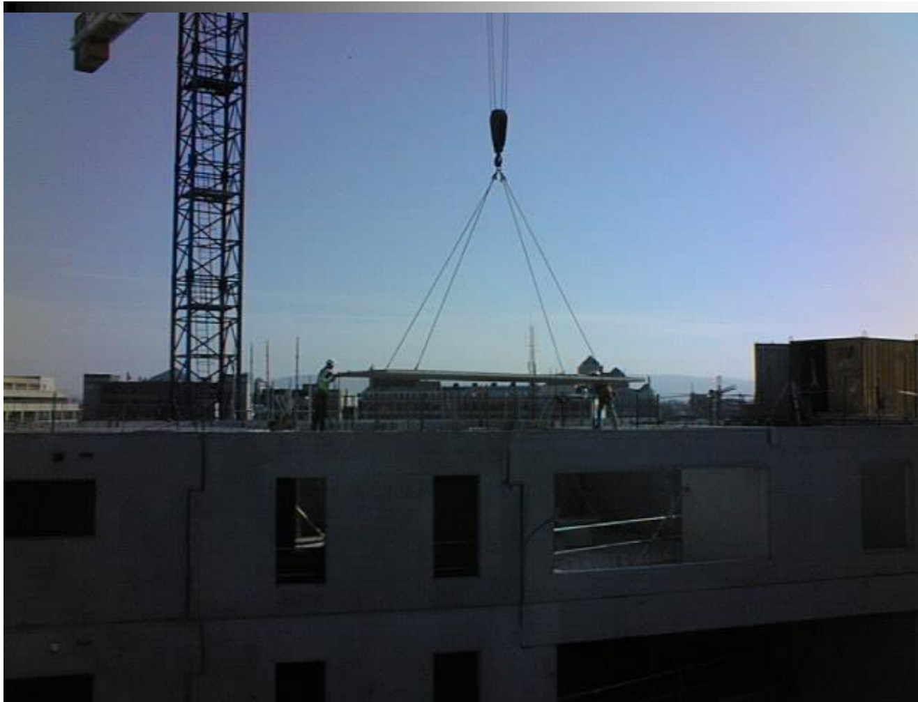
Precast floor panels, Dublin (Smallwood, 2004)
