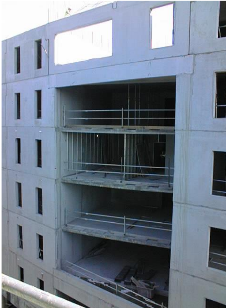
Precast wall panels, Dublin (Smallwood, 2004)
