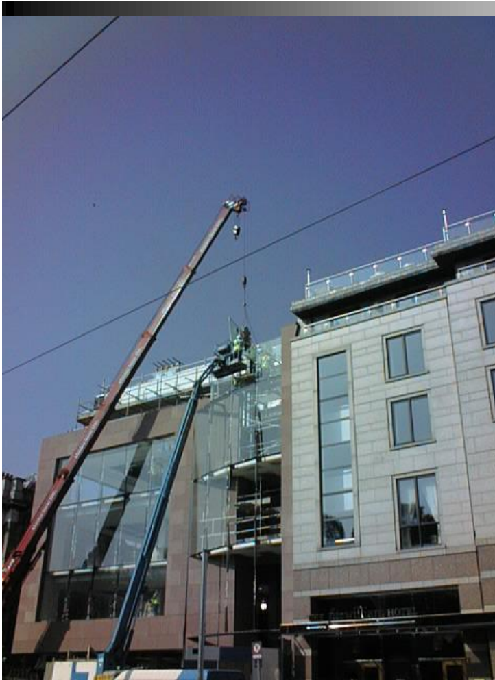
Externally installed full fenestration, Dublin (Smallwood, 2004)
