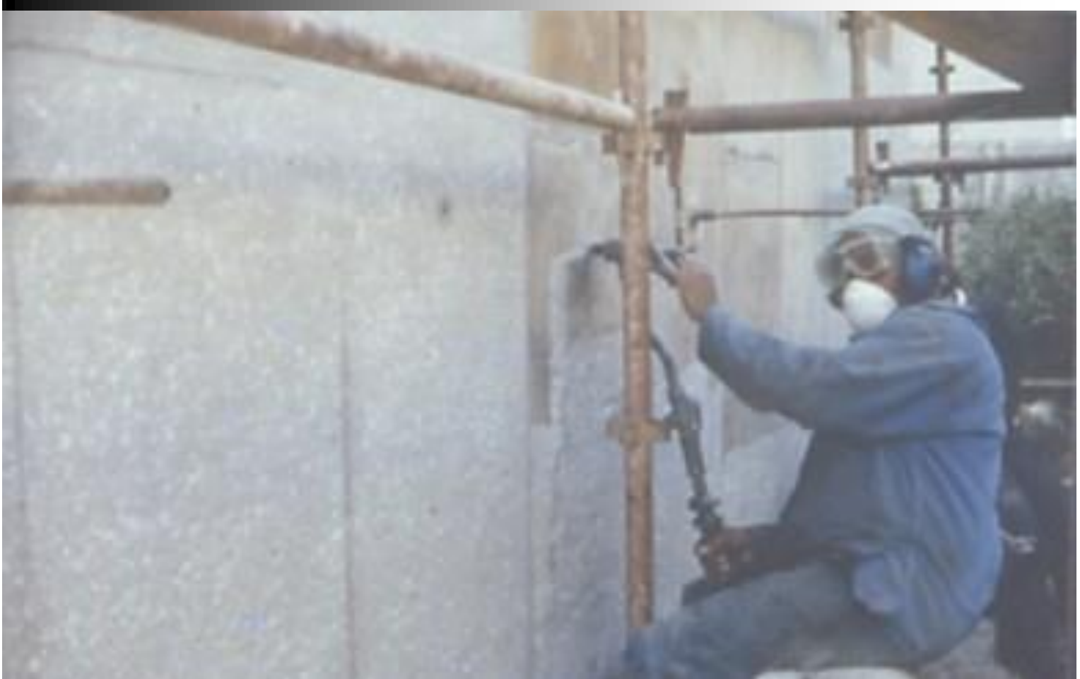
Bush-hammered concrete, UPE (Smallwood, 1994)
