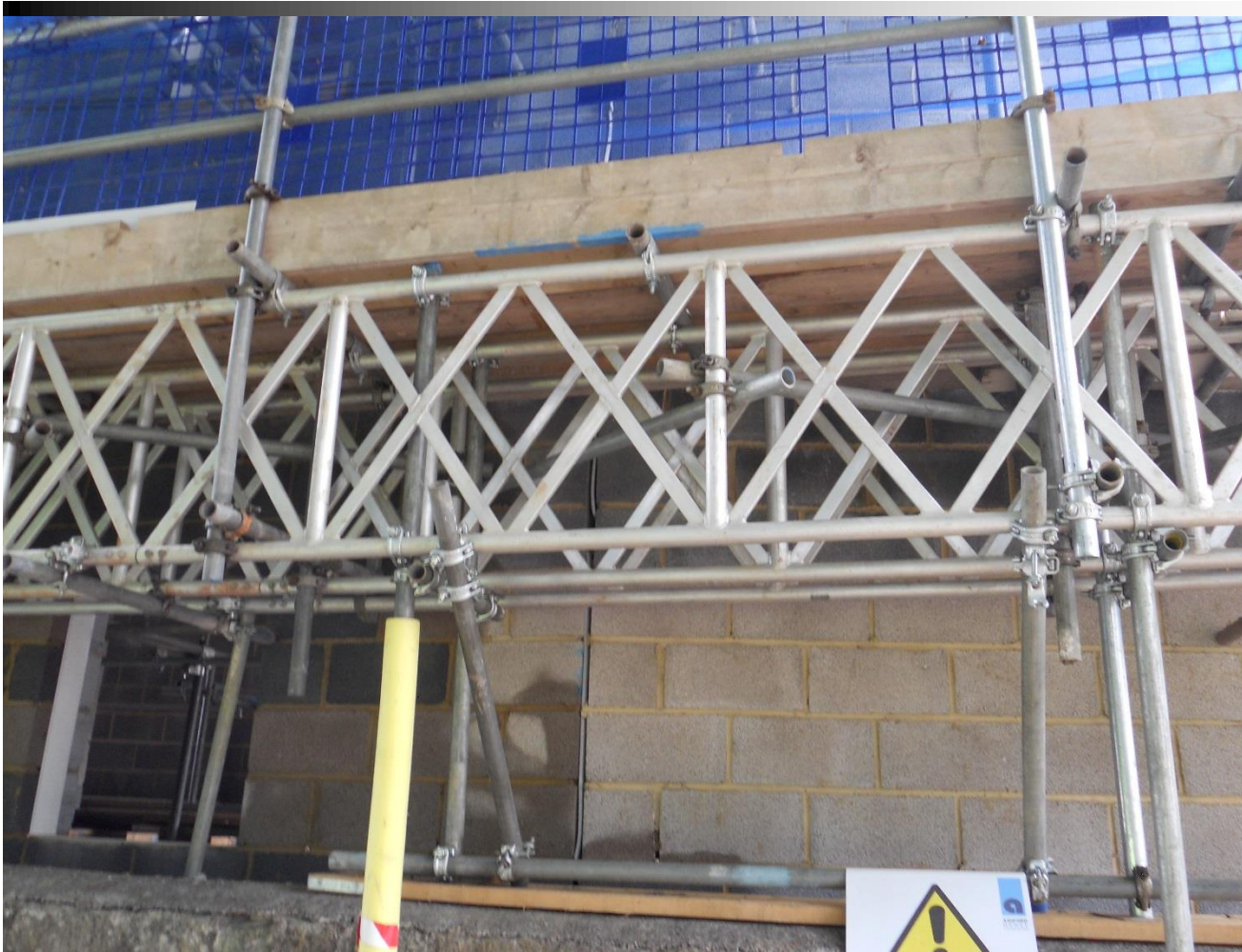
Scaffolding, Bradford on Avon (Smallwood, August 2014)
