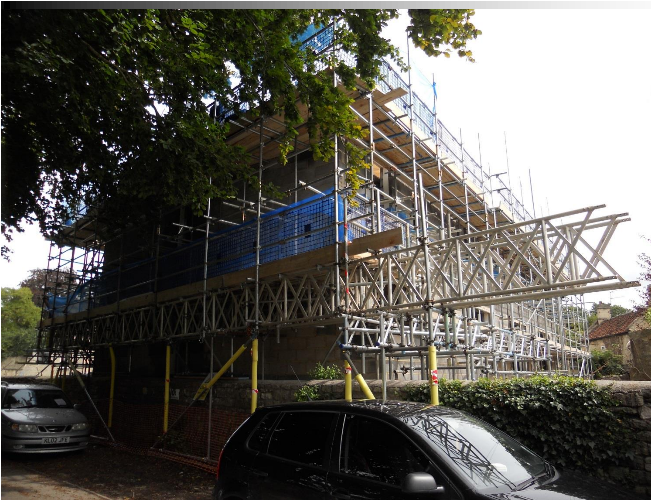
Scaffolding, Bradford on Avon (Smallwood, August 2014)
