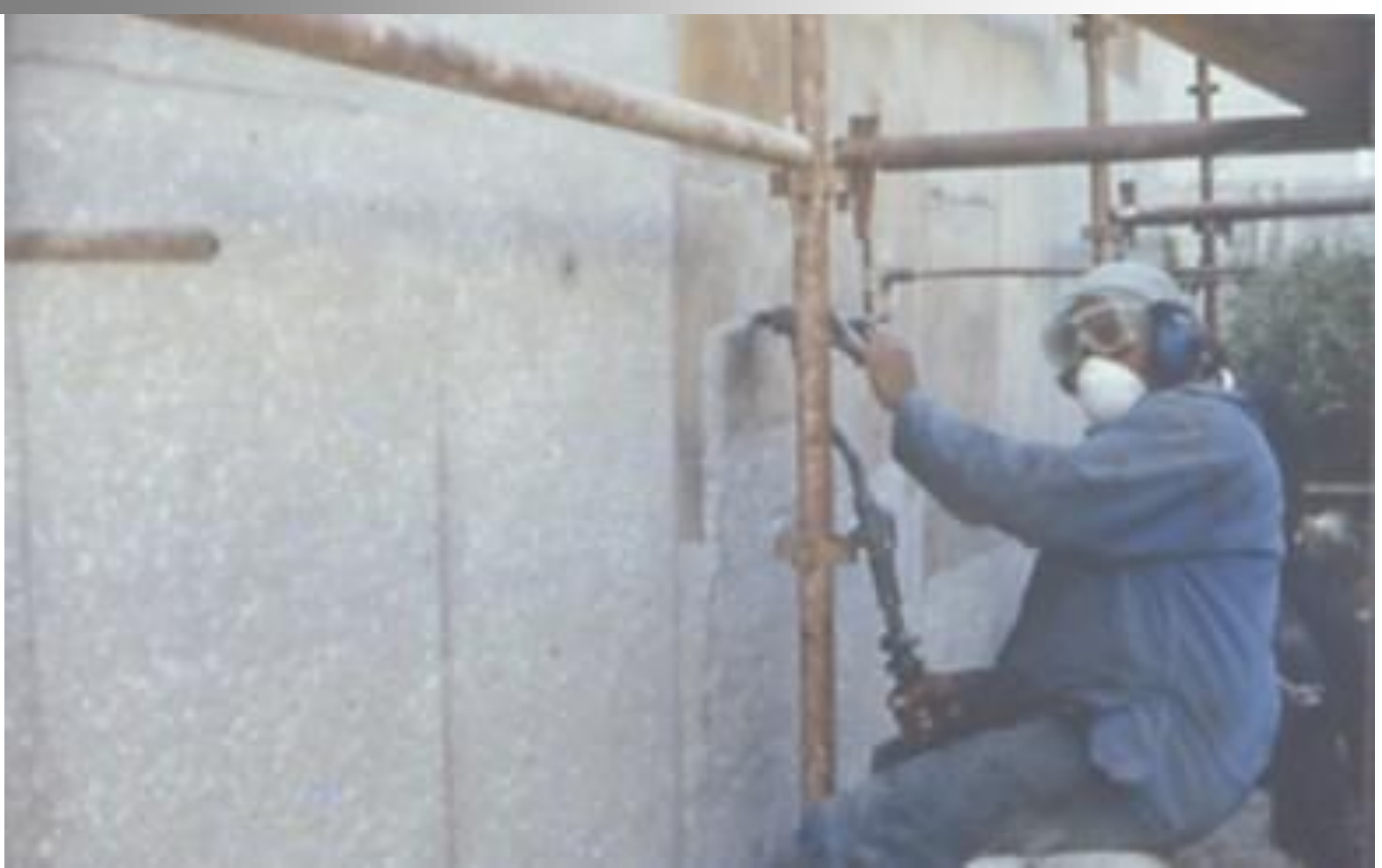
'Bush-hammered' concrete, Port Elizabeth (Smallwood)
