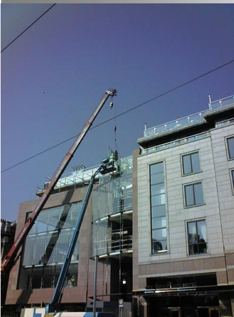
Externally installed full fenestration, Dublin (Smallwood, 2004)
