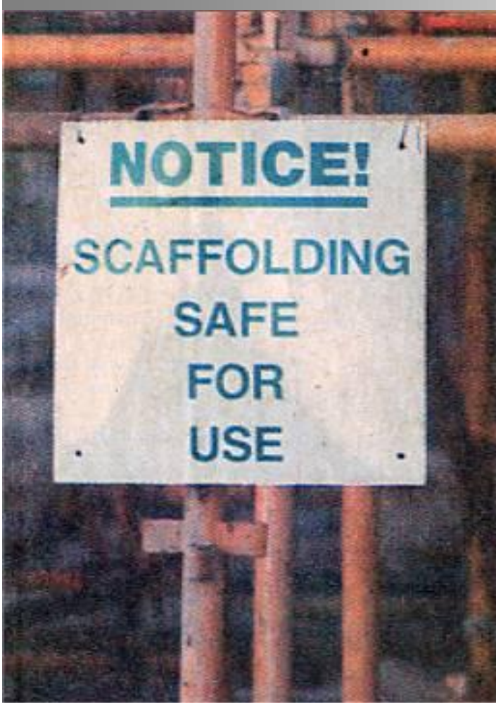
Coega Bridge collapse, Port Elizabeth, November, 2003 (Markman, 2003)
