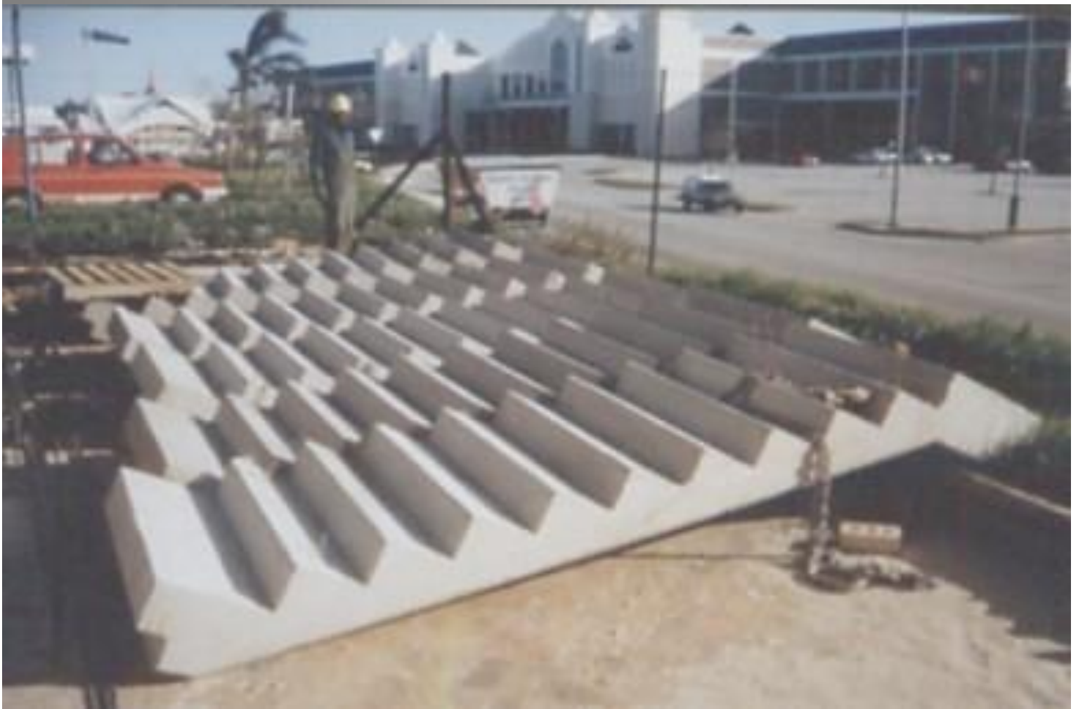
Precast concrete stair flights, Port Elizabeth (Smallwood)
