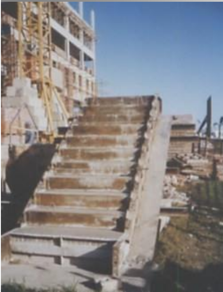
Precast concrete stair flights, Port Elizabeth (Smallwood)
