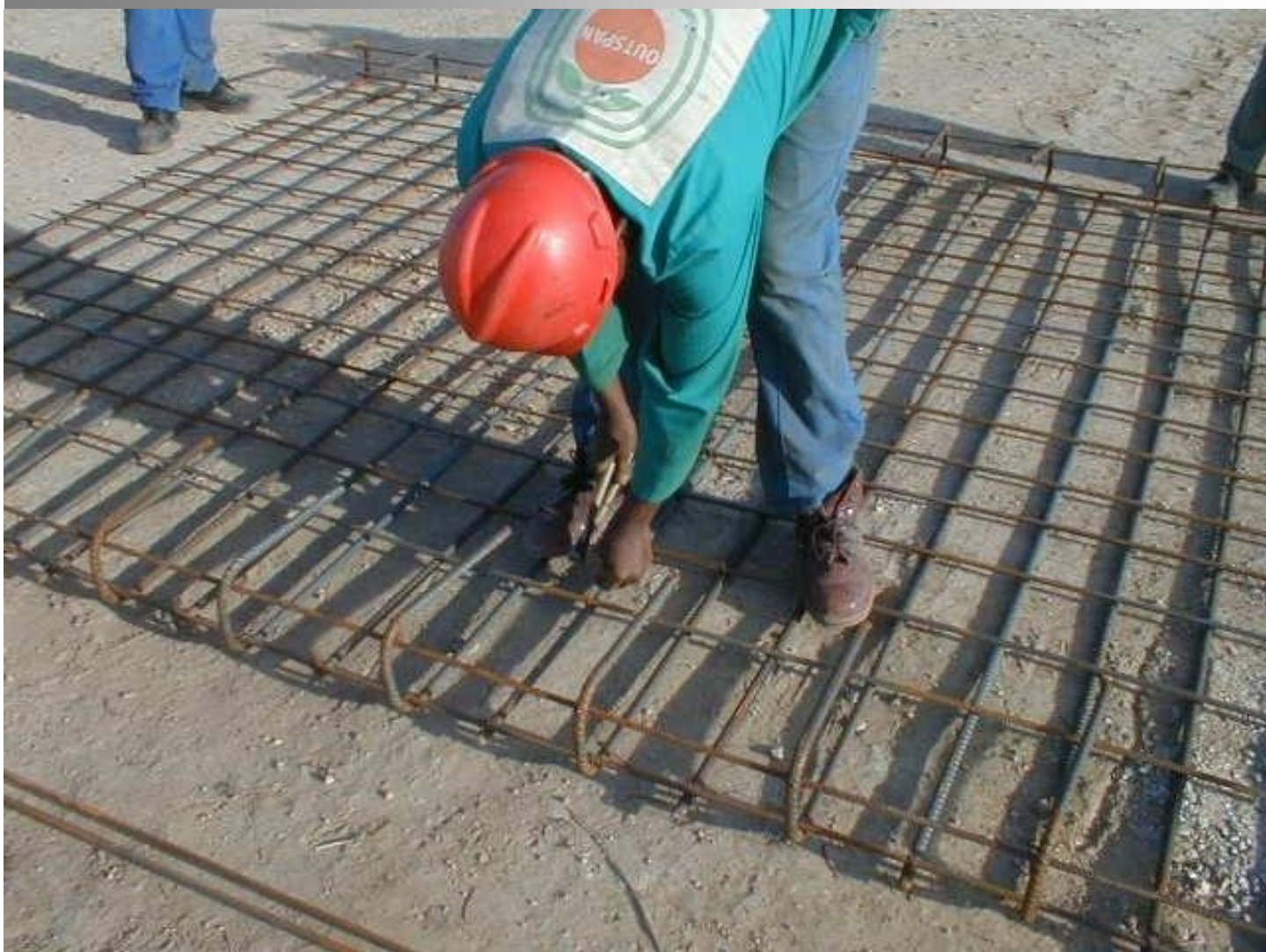
Tying reinforcing – bending, rapid repetitive movements etc. (Deacon, 2004)
