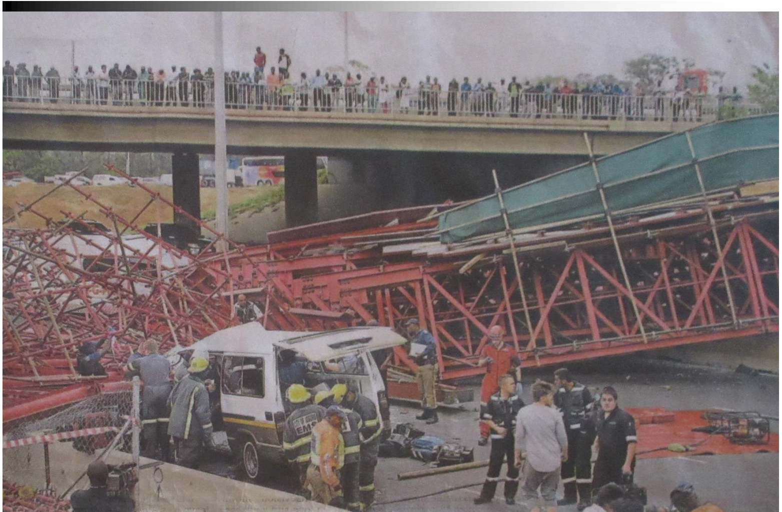
M1 Highway Temporary Bridge collapse, Johannesburg, 14 October 2015 (Reuters)
