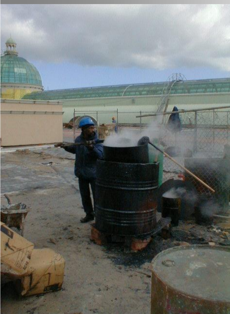
'Melting' mastic asphalt, Canal Walk, Cape Town (Smallwood, 2000)
