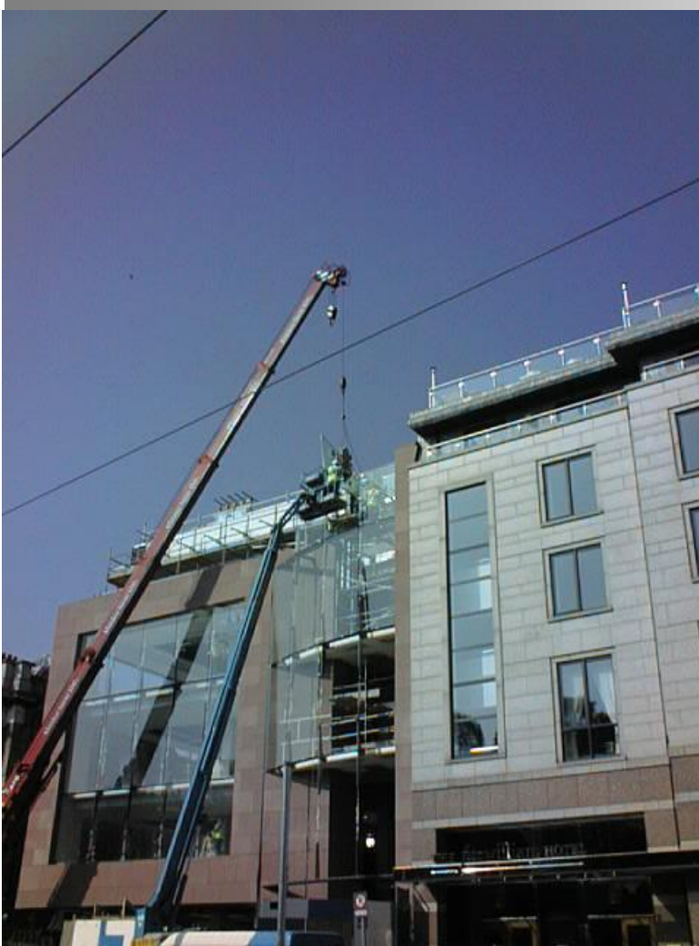
Externally installed full fenestration, Dublin (Smallwood, 2004)
