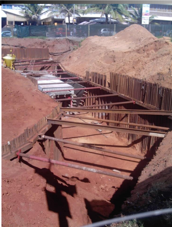
Culvert construction within a trenched sheeted excavation, Umhlanga (Smallwood, 2007)
