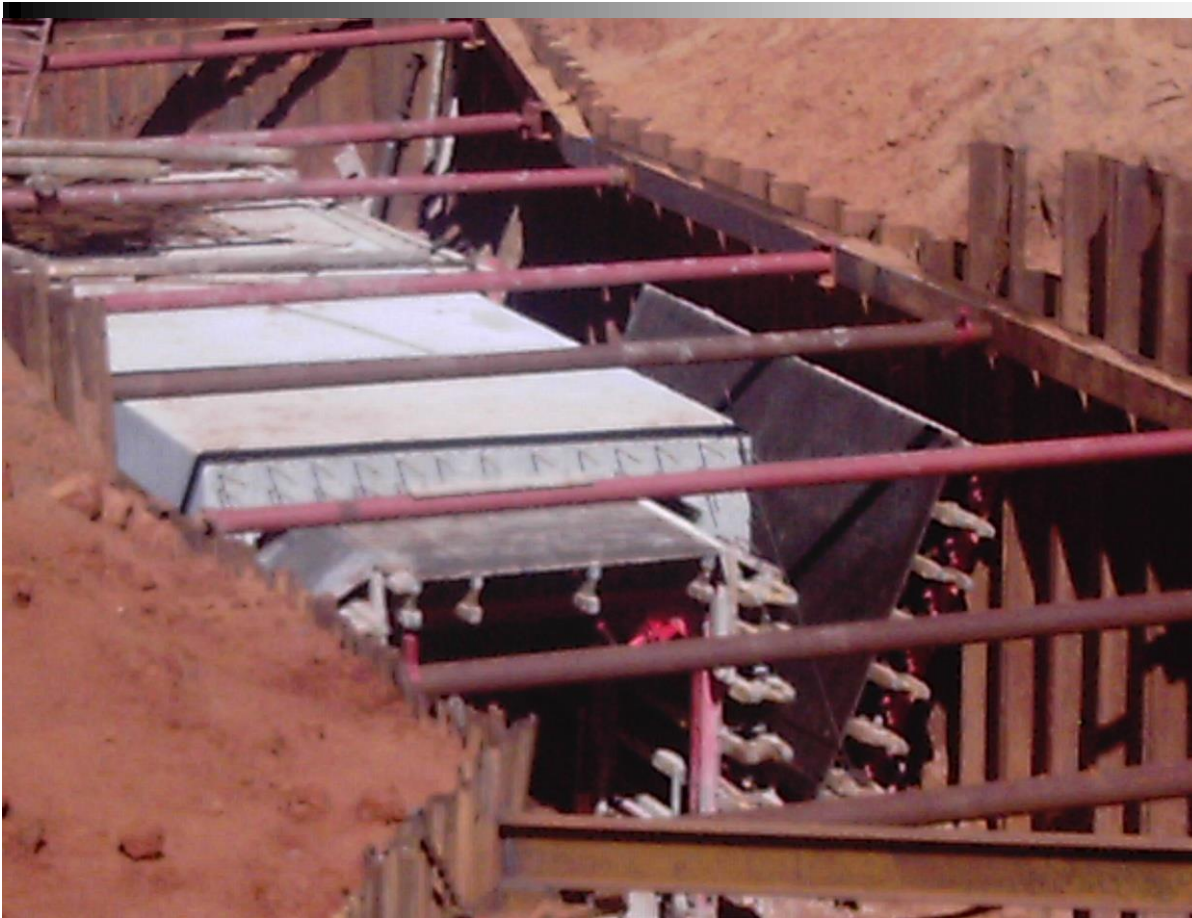
Culvert construction within a trenched sheeted excavation, Umhlanga (Smallwood, 2007)
