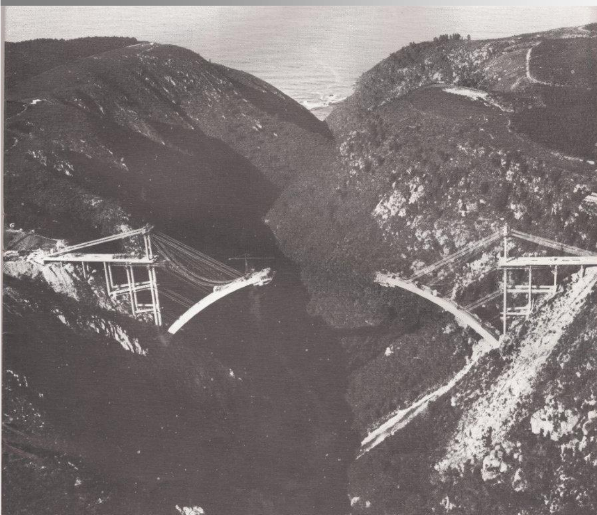
Bloukrans Bridge (p. 11, Concrete Beton, 1983)
