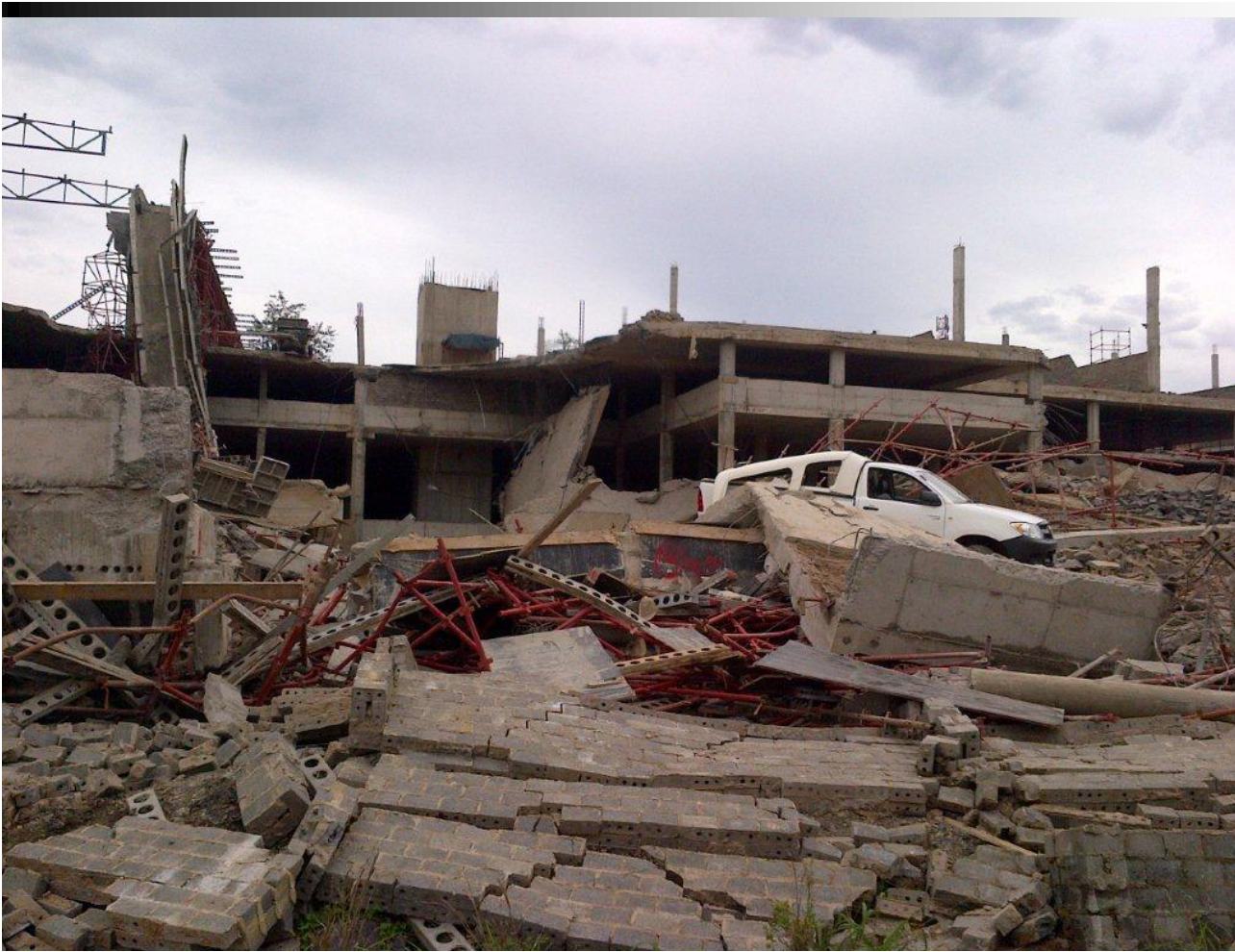
Tongaat Mall Collapse, 19 November 2013
