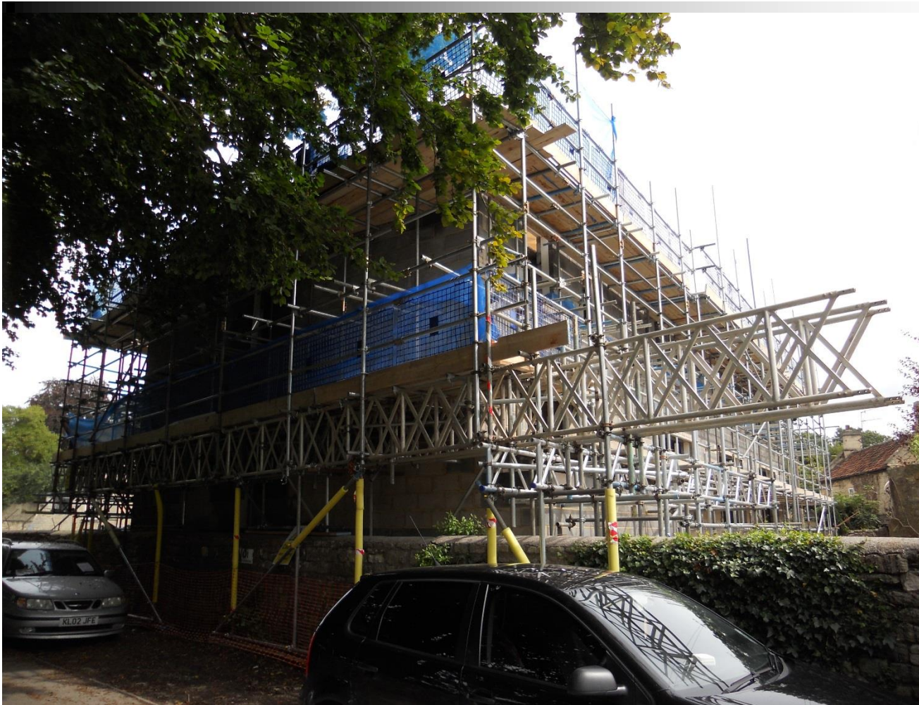
Scaffolding, Bradford on Avon (Smallwood, August 2014)
