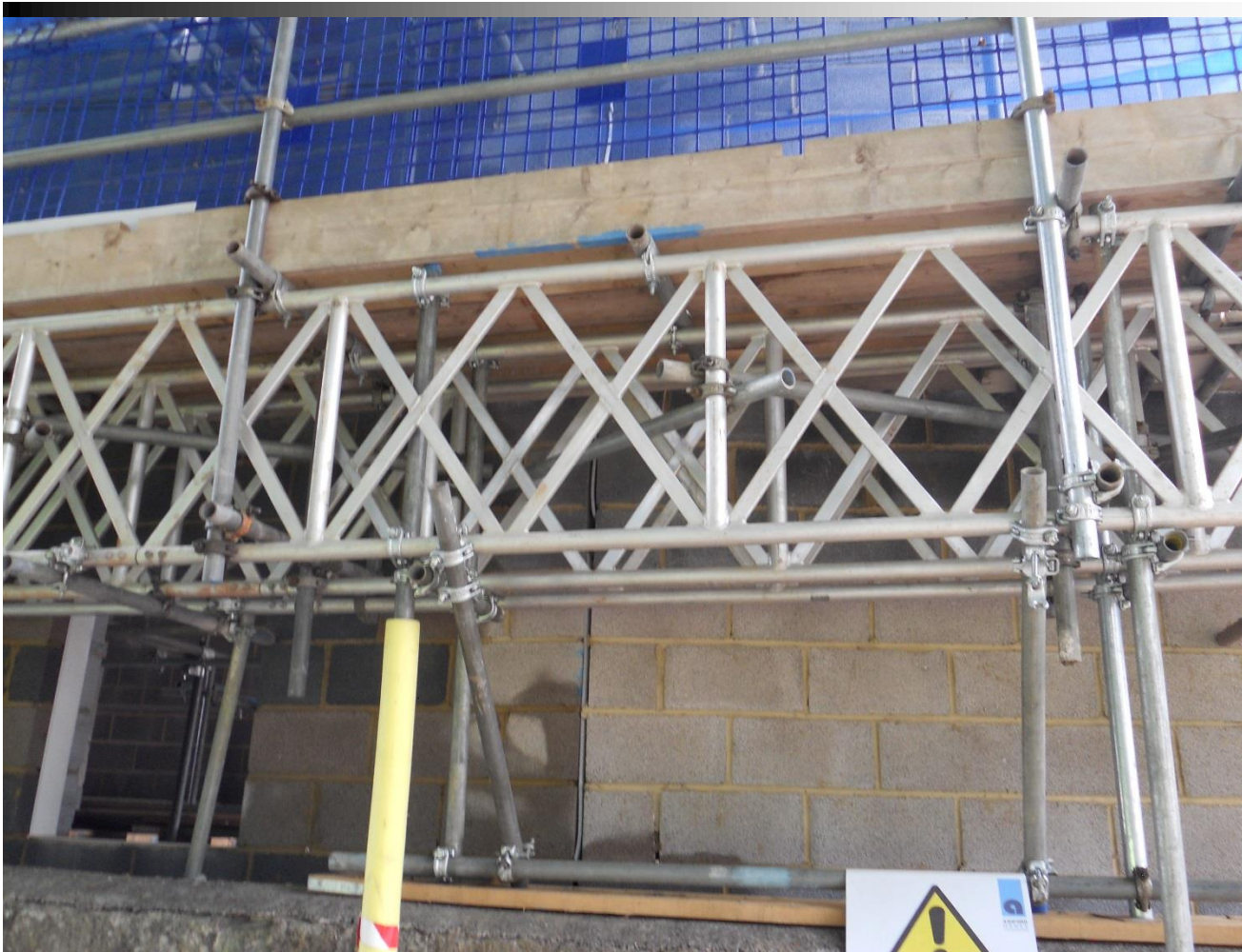
Scaffolding, Bradford on Avon (Smallwood, August 2014)
