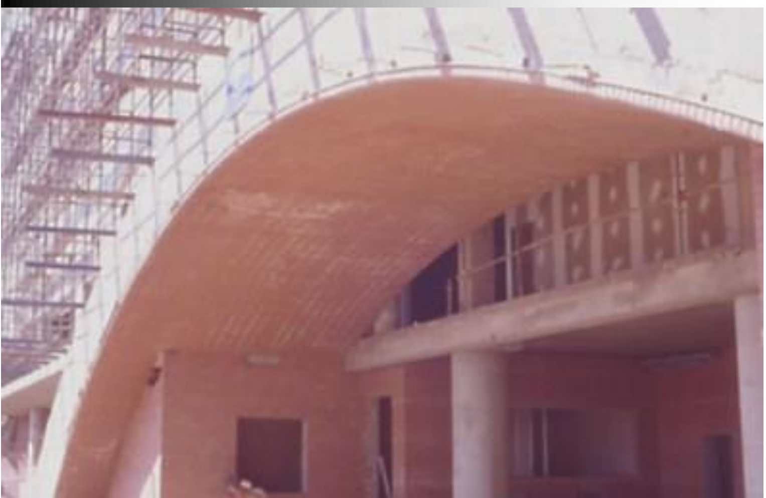
Face brick lining to semi-circular RC soffit, Sandton (Smallwood)
