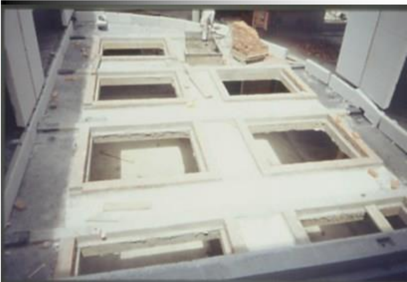
Natural-light openings, Port Elizabeth (Smallwood)
