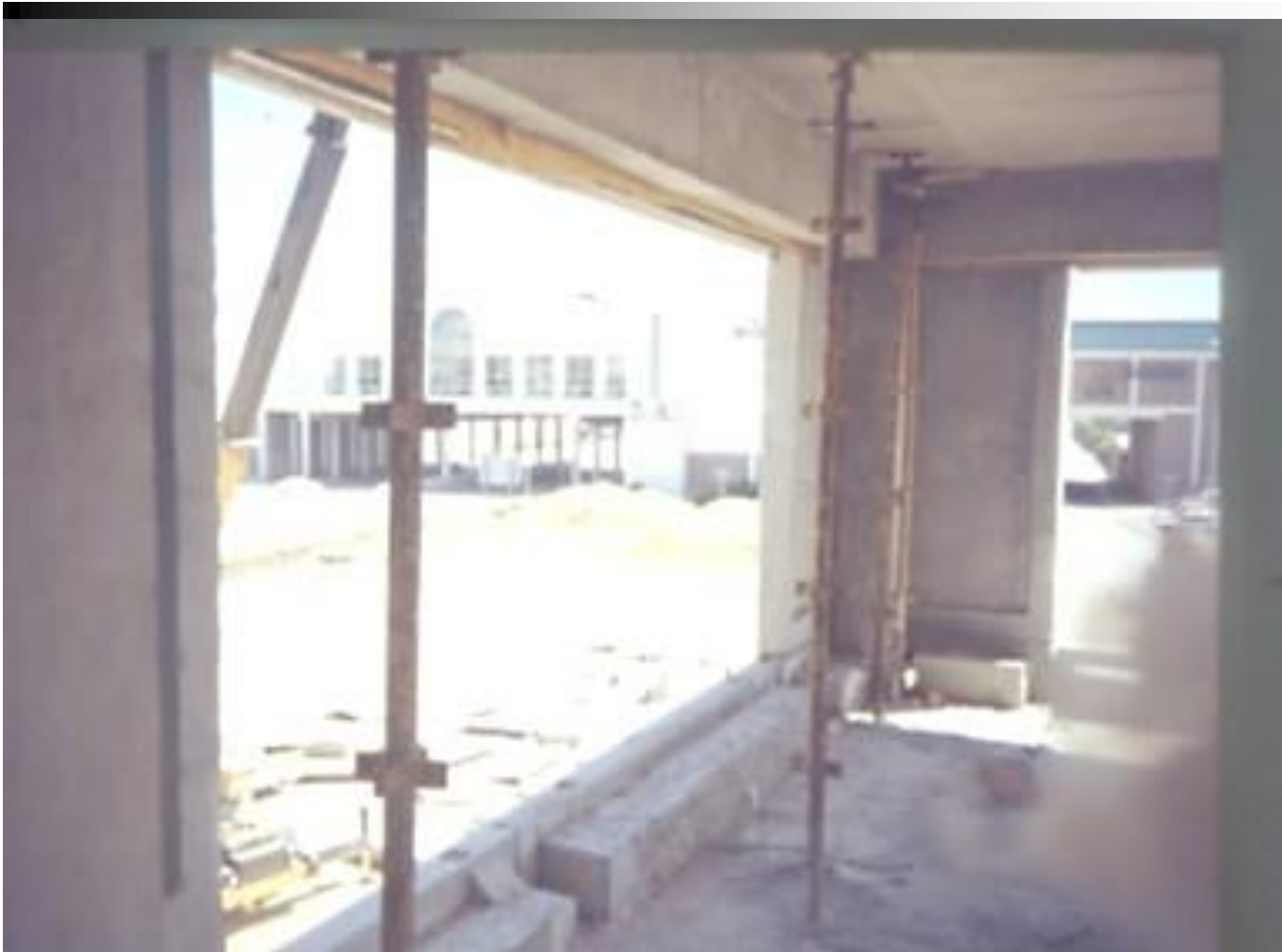
'Open' precast concrete cladding, Port Elizabeth (Smallwood)
