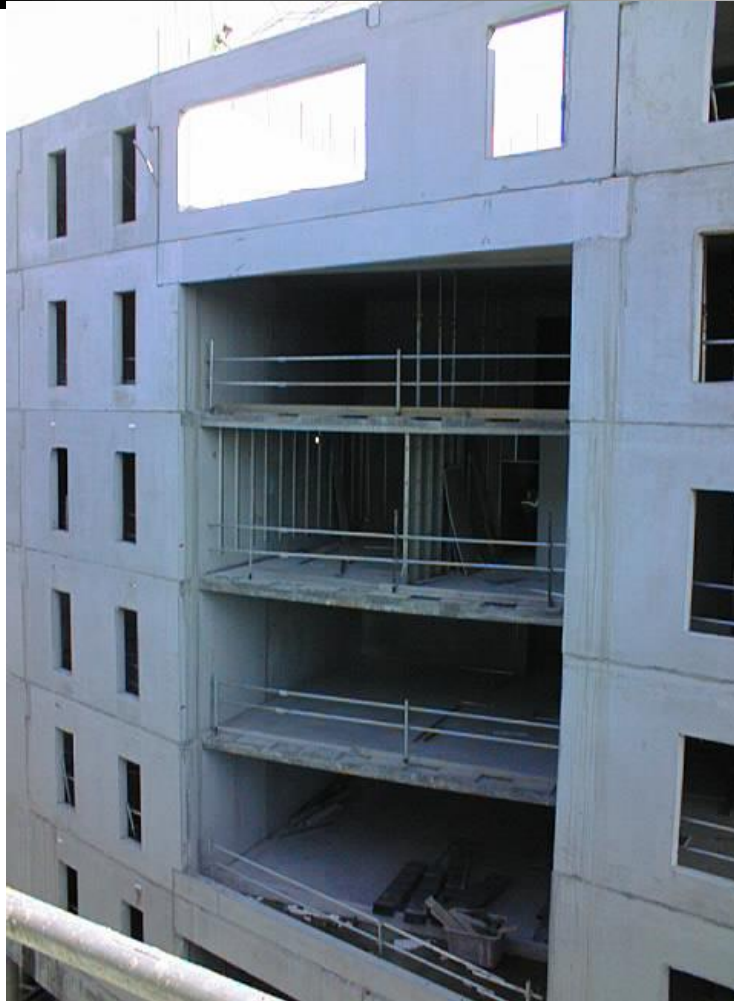
Precast wall panels, Dublin (Smallwood, 2004)
