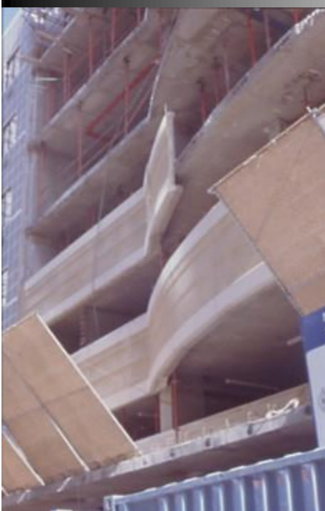
'Balustrade' precast concrete cladding, Cape Town (Smallwood)
