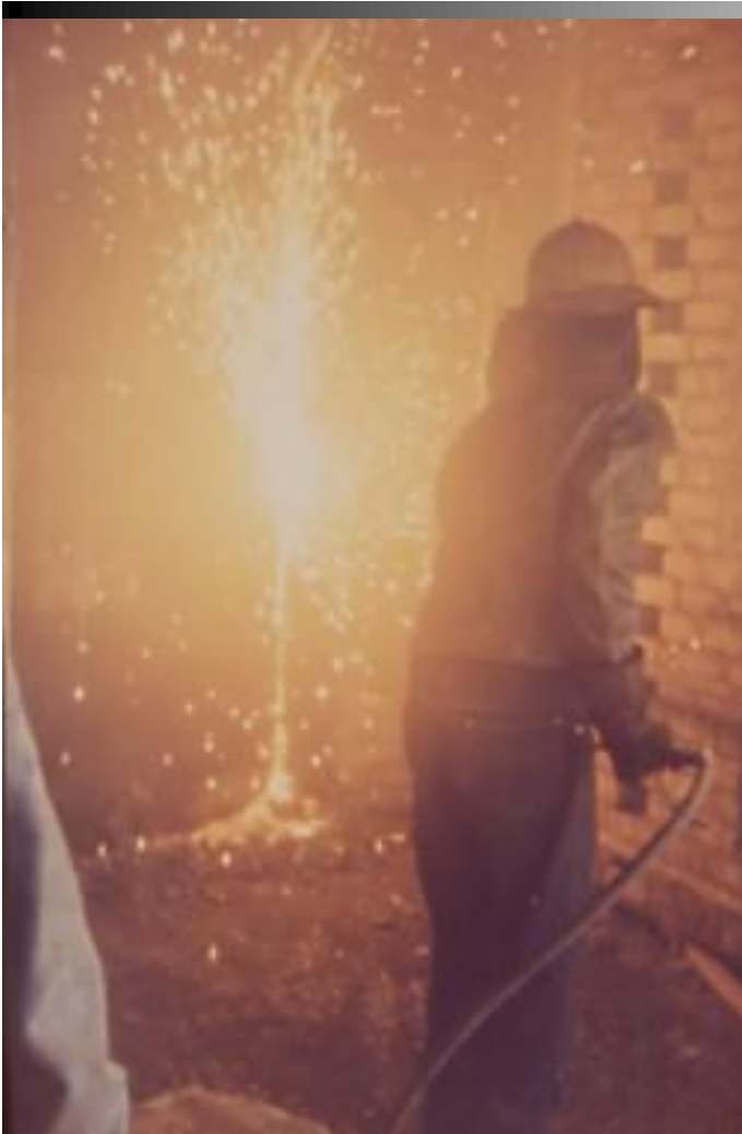
Thermal Lance, Mount Road Police Station, Port Elizabeth (Smallwood, 1987)
