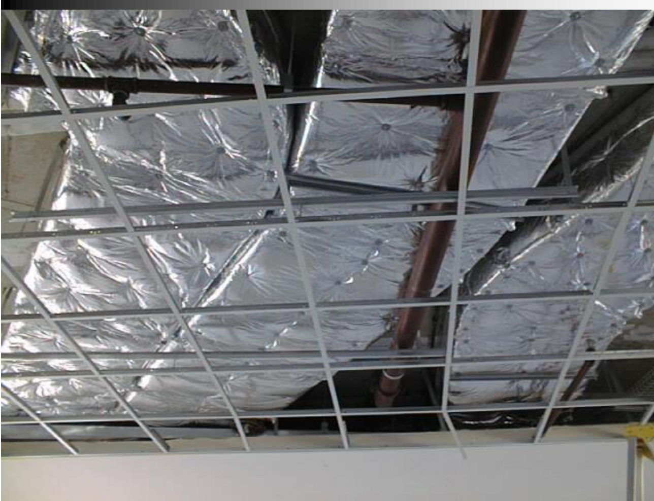
Congested ceiling space, Cape Town (Smallwood, 2004)
