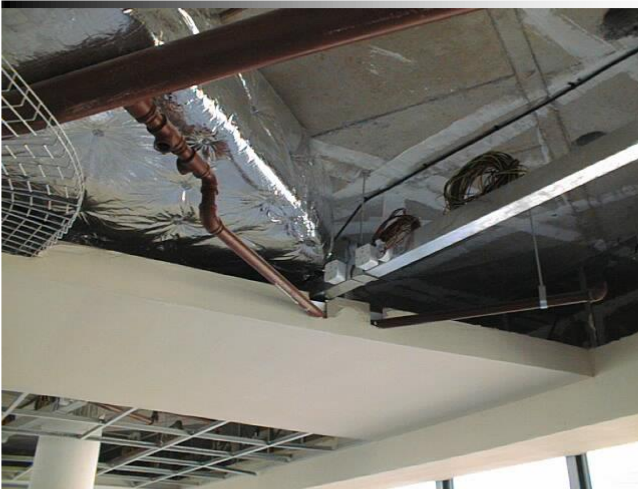
Congested ceiling space, Cape Town (Smallwood, 2004)
