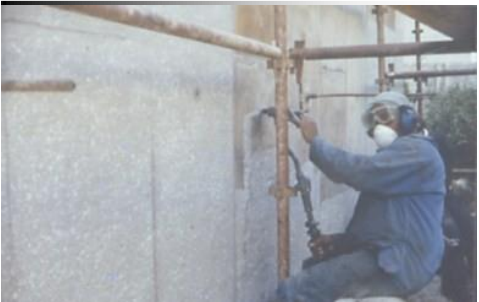
'Bush-hammered' concrete, Port Elizabeth (Smallwood)
