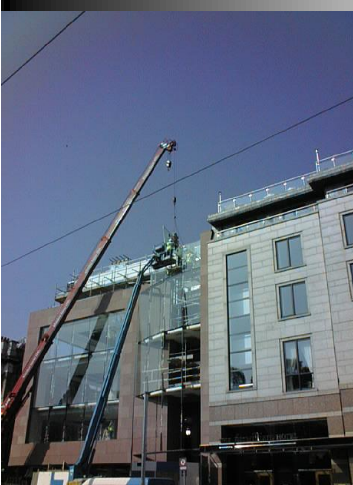
Externally installed full fenestration, Dublin (Smallwood, 2004)
