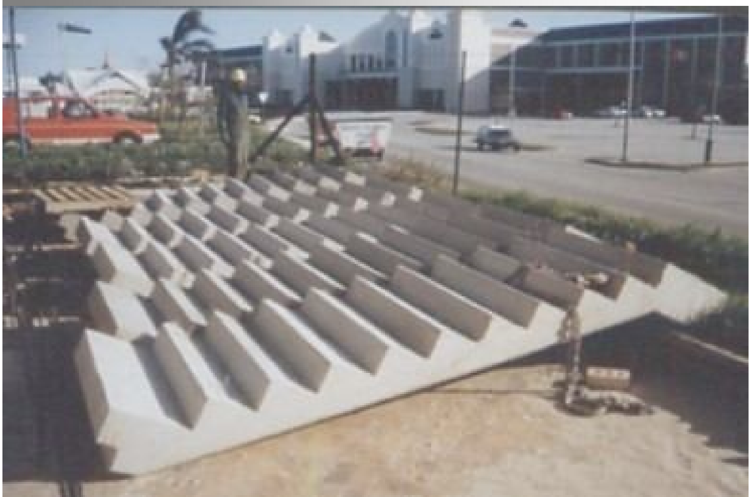
Precast concrete stair flights, Port Elizabeth (Smallwood)
