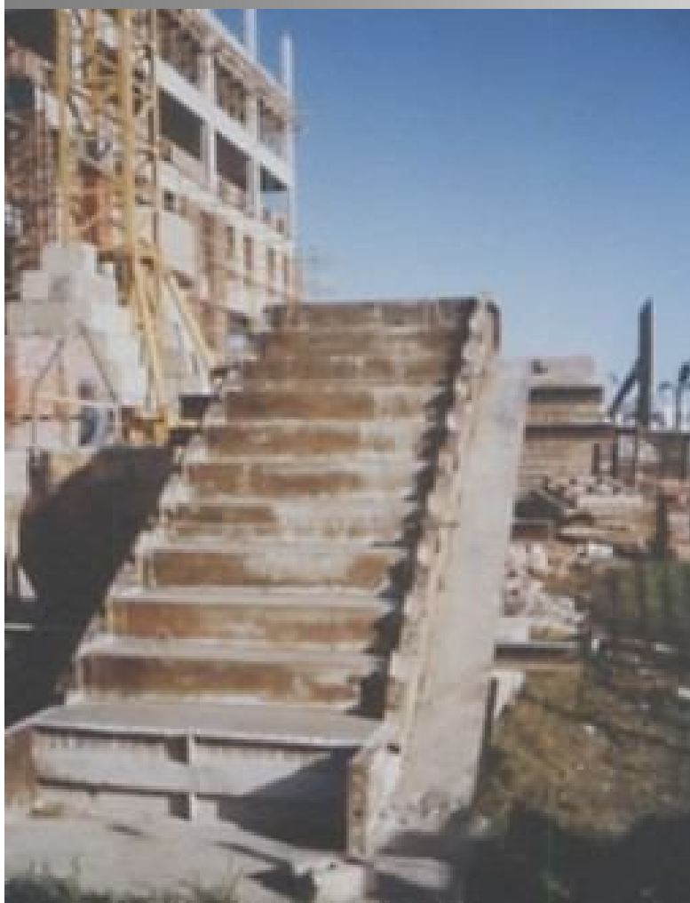
Precast concrete stair flights, Port Elizabeth (Smallwood)
